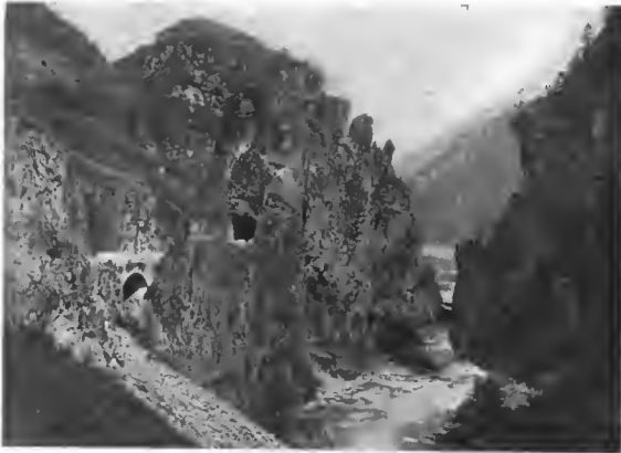
Where St. Gothard Pass Becomes a Pitch Black Tunnel.
